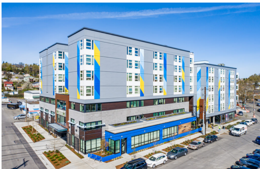
DESC Hobson Place. Photo credit: Walsh Construction Co.
